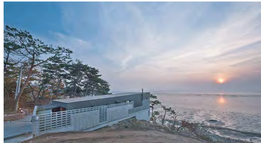
DETACHED HOUSE IN GANGHWA 강화 단독주택
